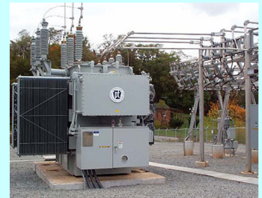
Power feed substation
