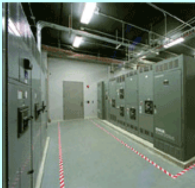
Transfer panel switch
