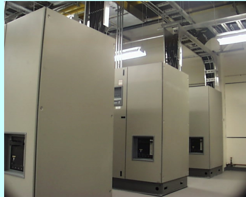
Uninterruptible Power Supply (UPS) modules
