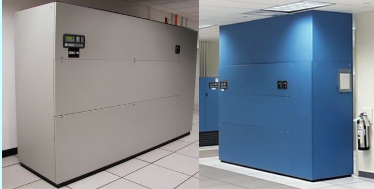
Computer Room Air Conditioning (CRAC) units
