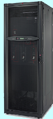
Power Distribution Unit (PDU)
