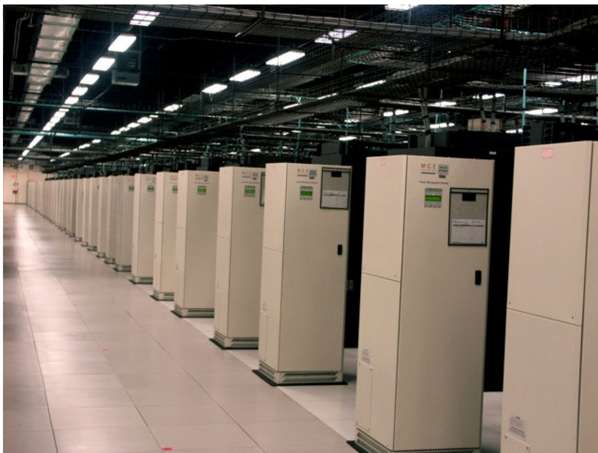
Power Distribution Units in a Data Center
